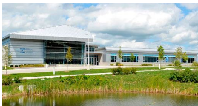
Figure 8: Walkerton Clean Water Centre
