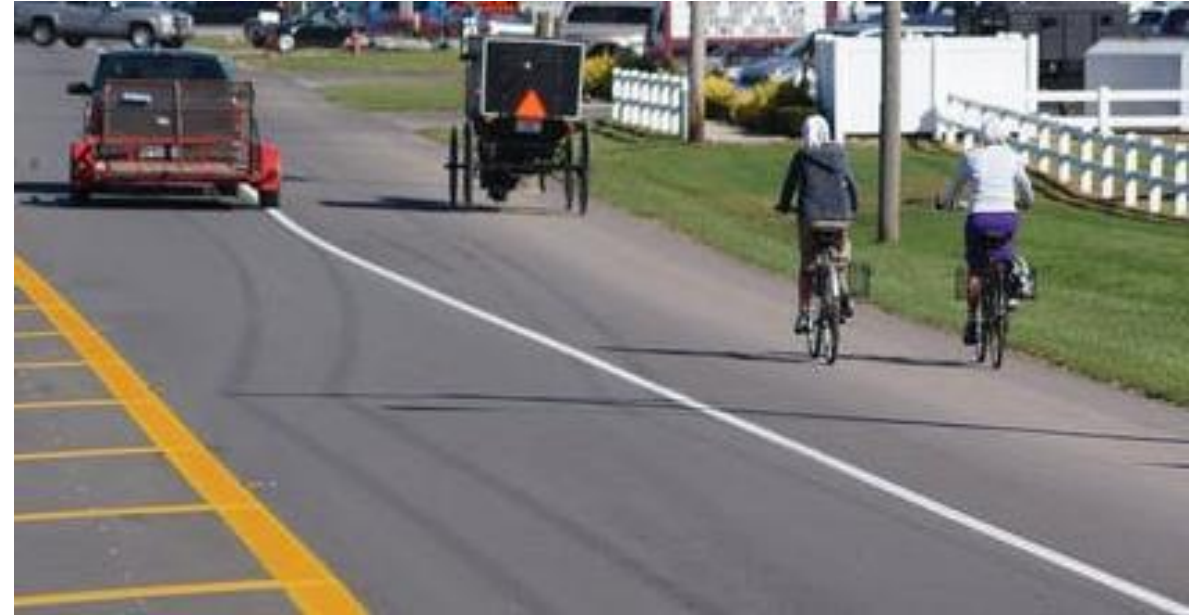
Example of a paved shoulder accommodating buggies and cyclists
