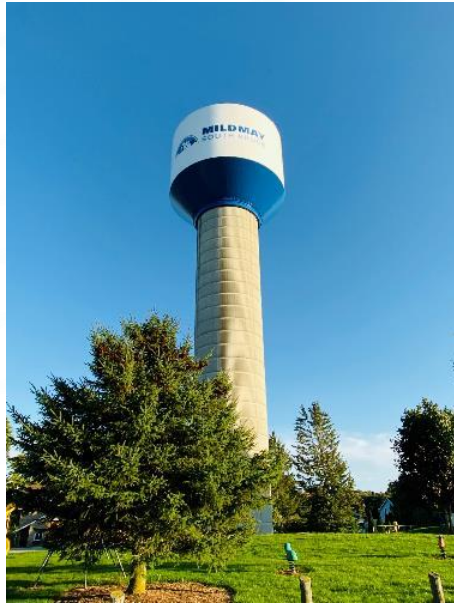
Potable Water Supply
