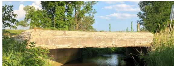
Structure 0021 on Sideroad 1A
