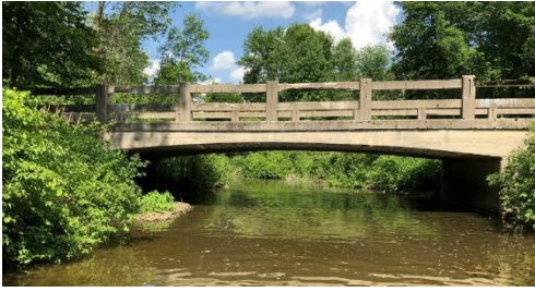
Structure 0019 on Sideroad 18
