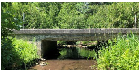
Structure 1019 on Sideroad 35
