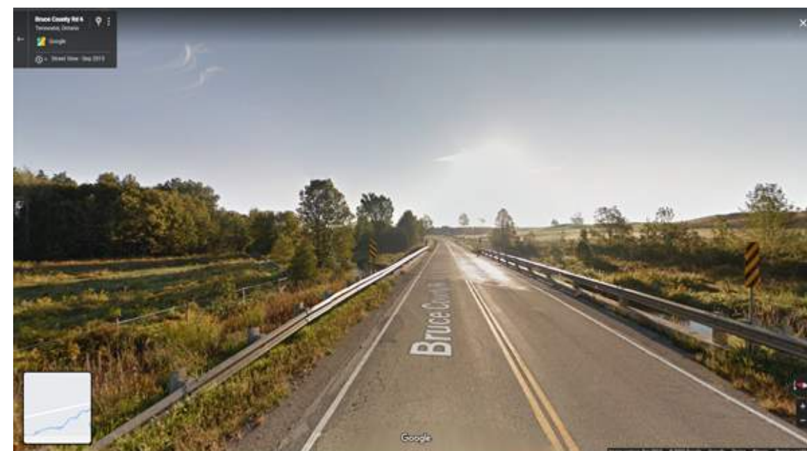
Figure 4. Watercourse Crossing - Forcemain/watermain to be installed using trenchless methods or supported on bridge
