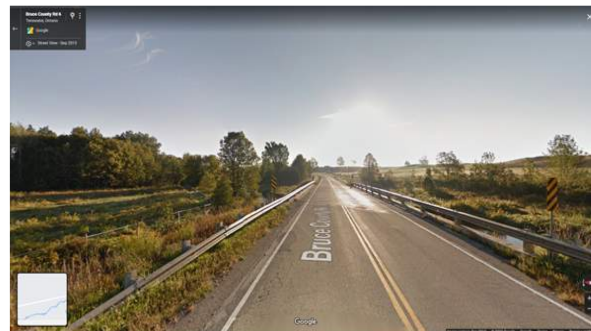
Figure 4. Watercourse Crossing - Forcemain/watermain to be installed using trenchless methods or supported on bridge
