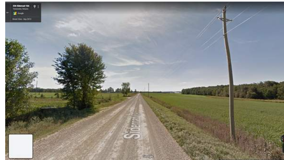
Figure D. Sideroad 10A - gravel surface minimized reinstatement cost
