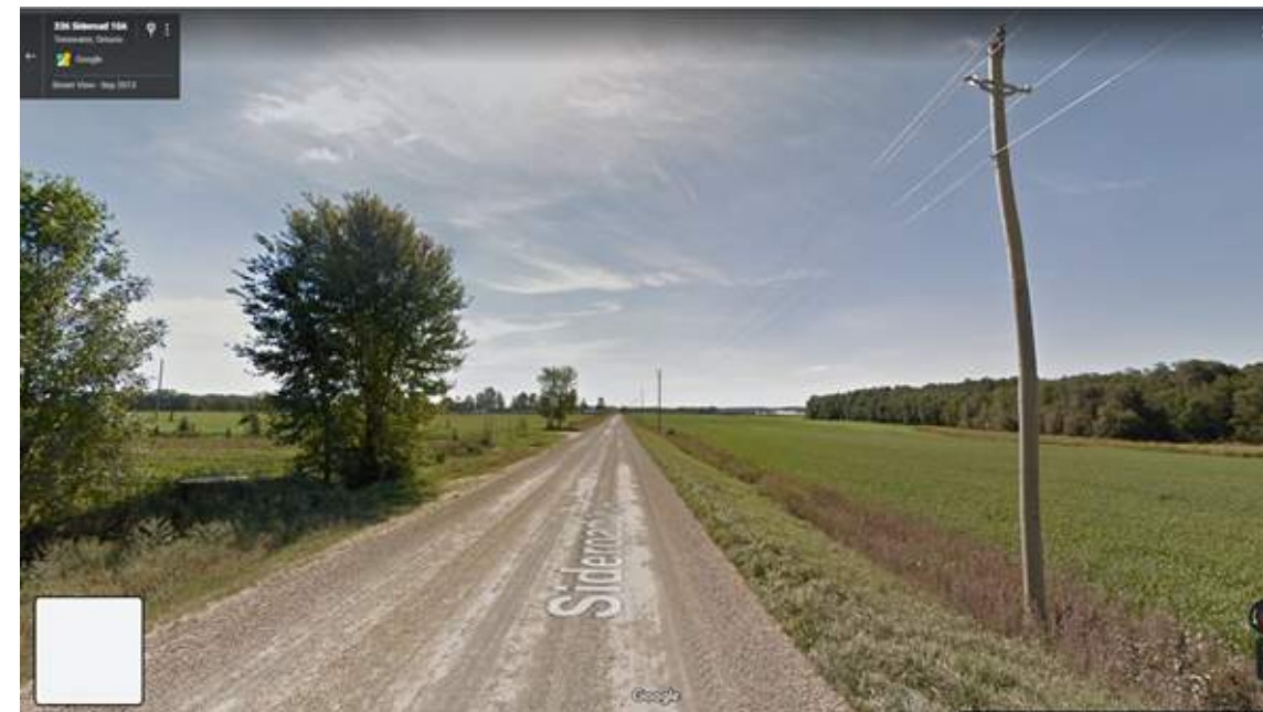
Figure D. Sideroad 10A - gravel surface minimized reinstatement cost
